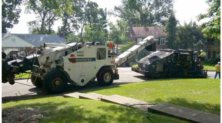
Workers apply nova chip surfacing to Nolan Drive.
