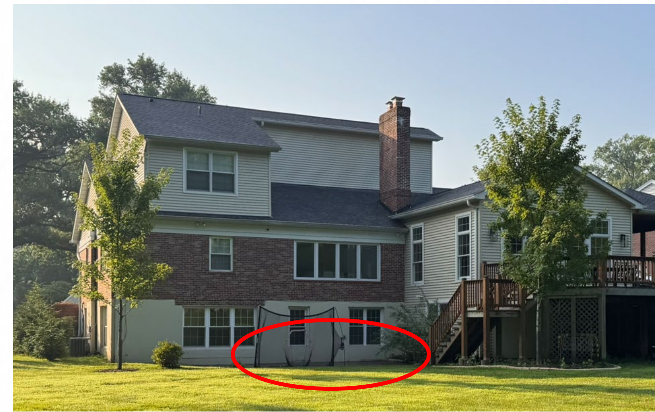
Walkout Basement Doors Replaced with Windows
